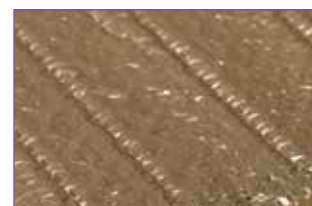
Unicell exterior face
